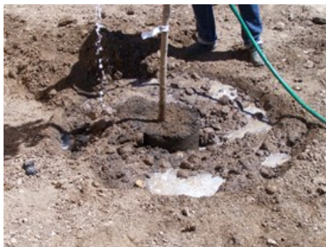
Watering tree during planting; notice how soil has settled.
